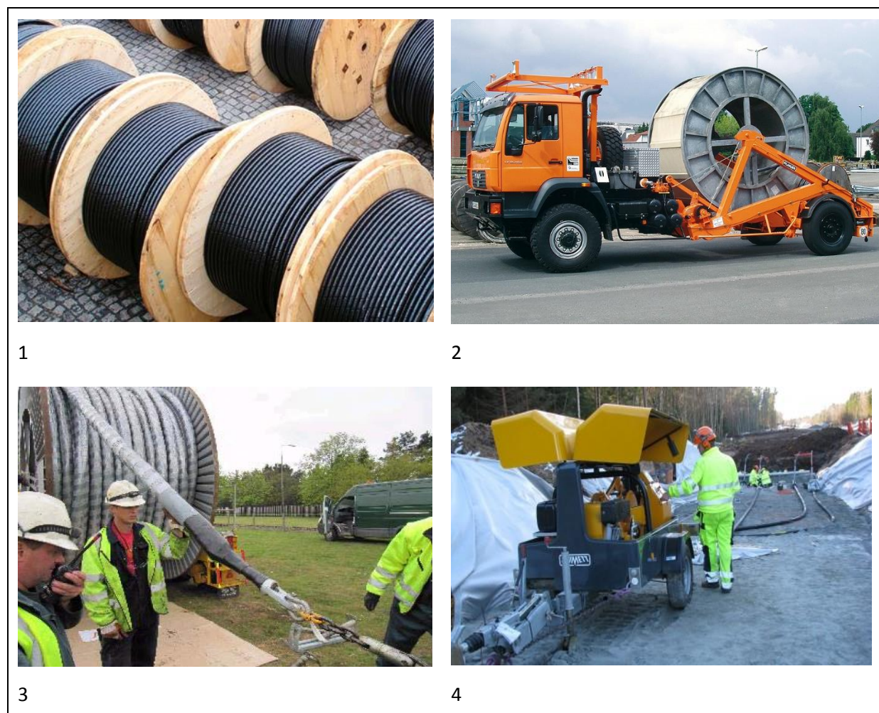
Figure 2.9. Exemplary 220 kV cable drums (1), vehicles with a cable trailer (2), LV cable winching operation (3), exemplary cable winch (4) [Source: okorder.com, lancier-cable.de, rampionoffshore.com, watucab.pl]
