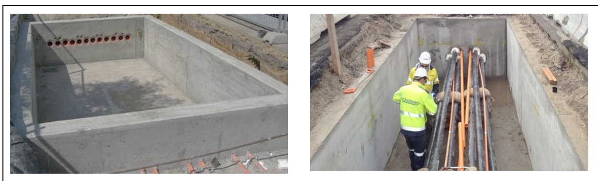
Figure 2.6. Exemplary cable chambers [Source: dunmain.com.au, sl-engineers.asia.com]
